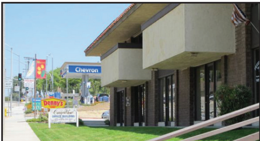
Canyon View Offices at 21308 Pathfinder Rd., Diamond Bar
