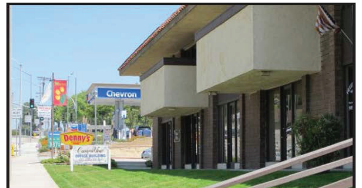
Canyon View Offices at 21308 Pathfinder Rd., Diamond Bar
