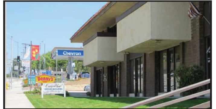
Canyon View Offices at 21308 Pathfinder Rd., Diamond Bar
